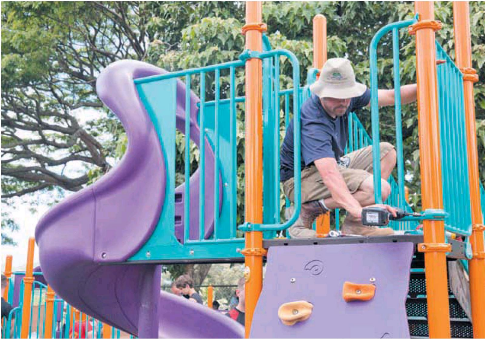
Todd Mazza helps assemble the 'rock-climbing' wall during Windward YMCA's marathon playground-building extravaganza May 25. Even Mickey and Minnie stopped by to watch the action. Photo by Rachel Breit, rbreit@midweek.com.
